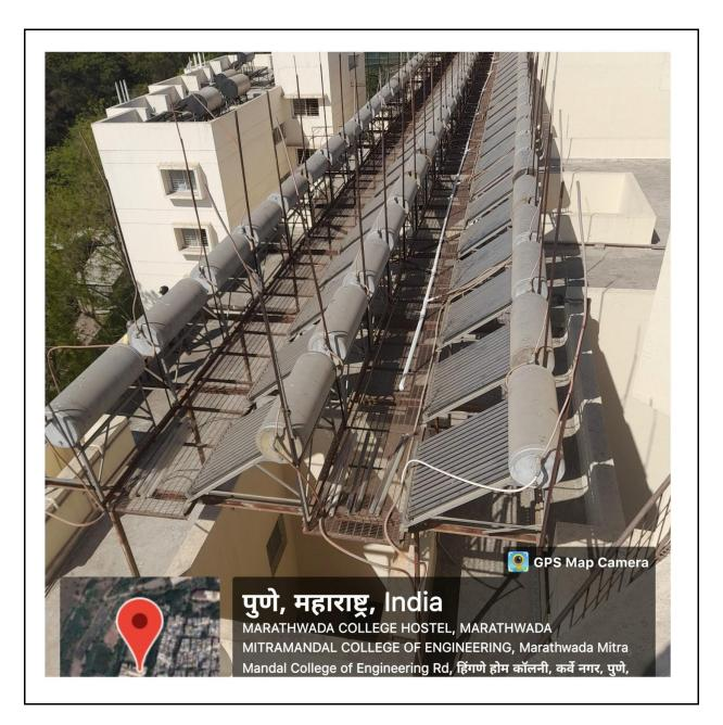
12750 litres per day (LPD) Solar Thermal Water Heating System
